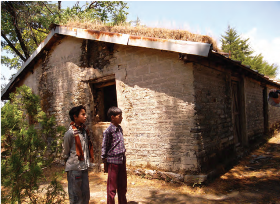
The old Kala Agar Forest Bungalow (erected 1925), where Corbett and the Vivians stayed (at different times) during the hunt of the Chowgarh man-eater. These two boys graciously guided us to this historic building in April 2012.
